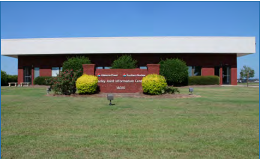
Plant Farley Joint Information Center
