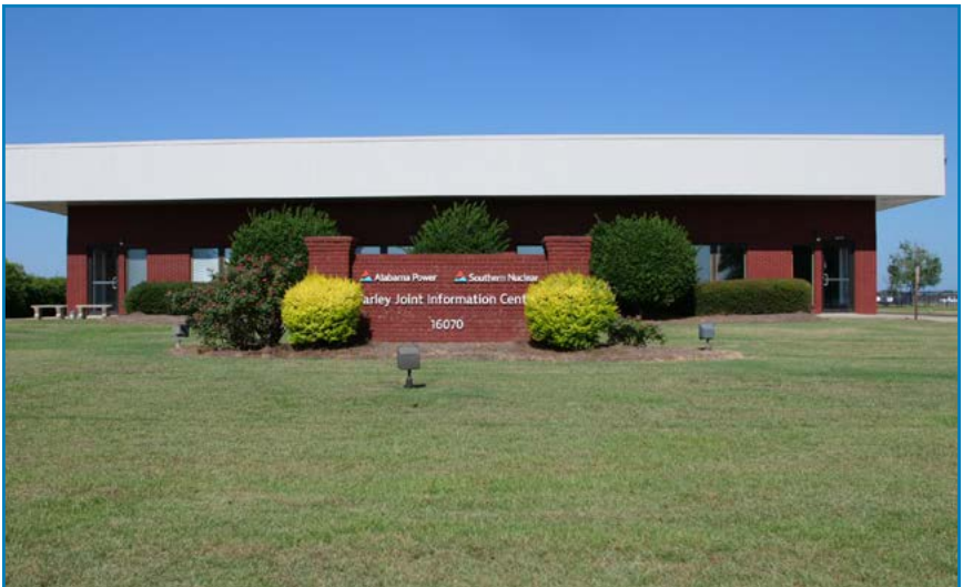
Plant Farley Joint Information Center
