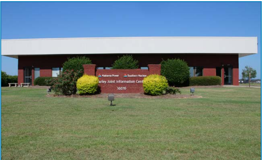
Plant Farley Joint Information Center
